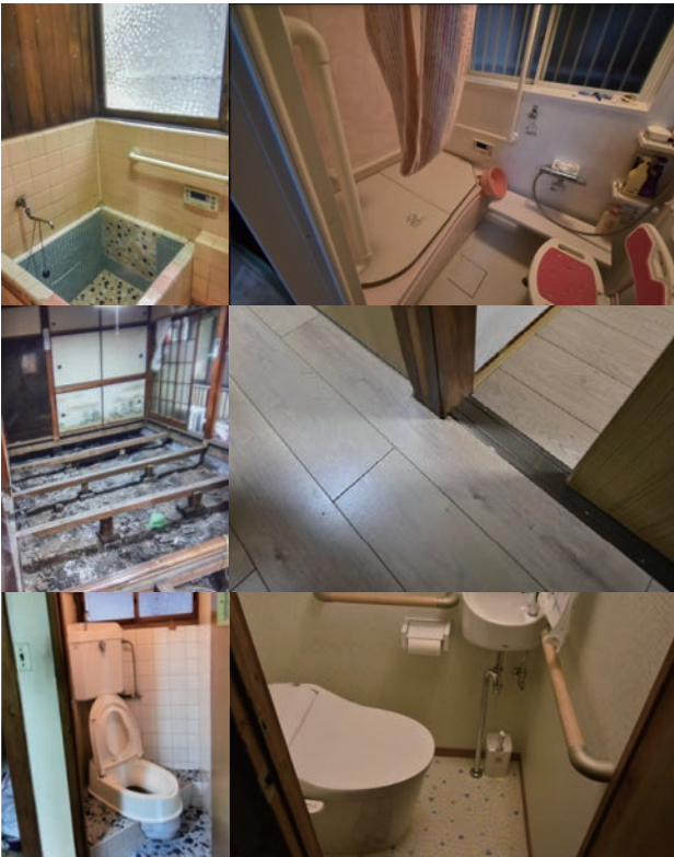
Fig. 3 Before(Left) & After(Right) Repair in No.4: Bathroom(Above), Living Room(Middle), Toilet(Bottom)
